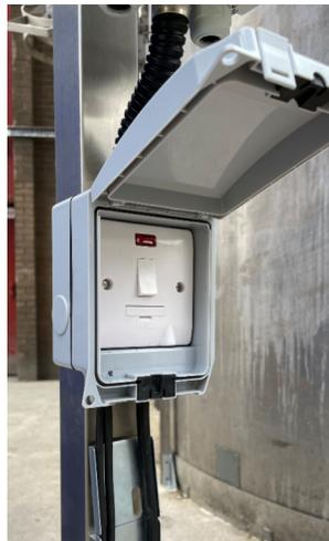
Lockable IP65 rated 3A fused spur protects circuit and allows for local isolation.
