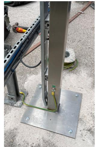
Metal plinth supplied with M8,0 earth point. Plinth mounted using four M10,0 rawl bolts.
